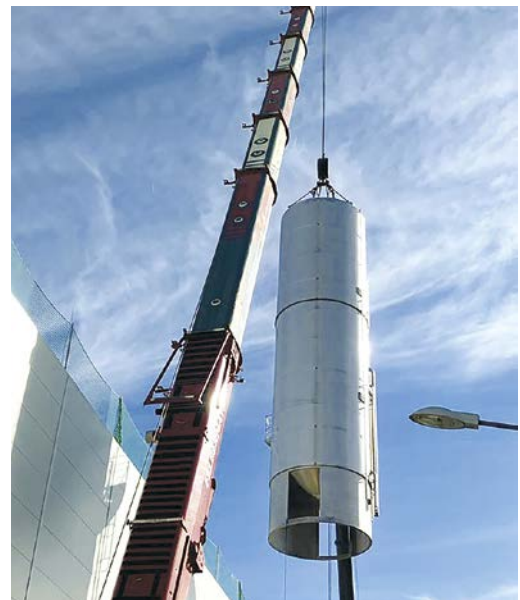
The new CIP tank has three chambers and a total volume of 120,000 liters (photo: Möstl)
