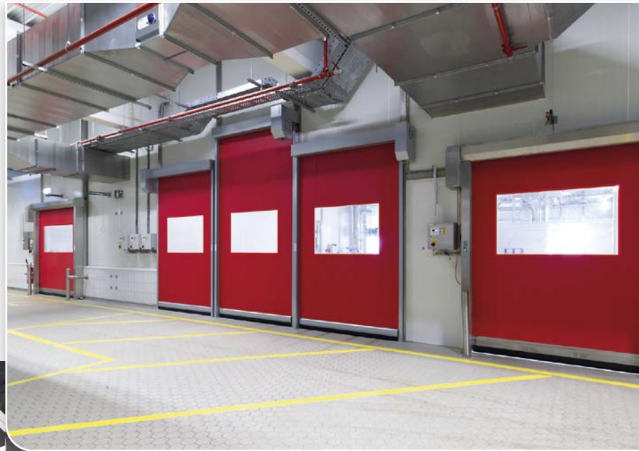
The doors open up to three times per minute, i.e. 180 times per hour (photo: EFAFLEX)
