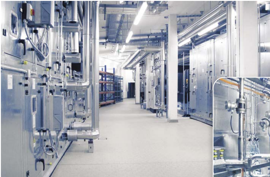
Central ventilation units in hygienic design with efficient heat recovery are part of the solution (photo: airinotec)
