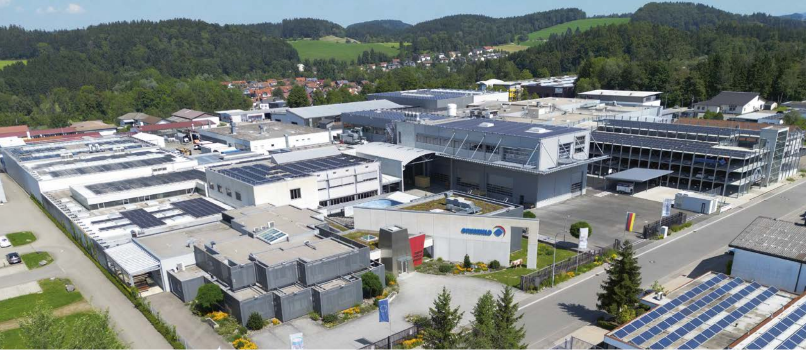
Aerial view of the GRUNWALD premises with the newly installed photovoltaic system with an output of 600 kWp (kilowatt peak) (photos: GRUNWALD)
